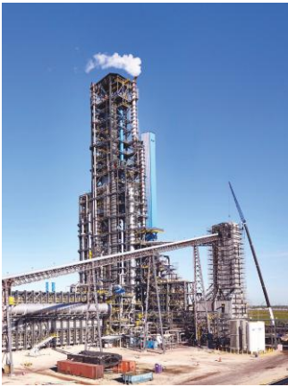
Fig.1: MIDREX Super MEGAMOD direct reduction shaft furnace in Corpus Christi, Texas. Source: Primetals Technologies primetals.com .
