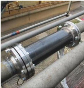
Fig.1: Sensor and signal processing unit installed at the main pipe for pulverized coal transport at voestalpine Linz. The pipe diameter is 150mm and operating temperatures are around 80°C (due to the pre-conditioning of the coal), thus temperature stability of the sensor and electronics is an important issue.
